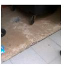
Floor damage, wheel catch/trip hazard
