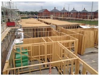
The crane has now been erected and construction of the timber frame has now commenced and is progressing at a rate of one floor a week.
