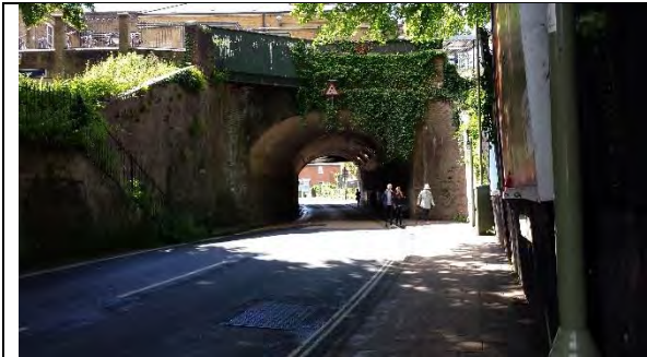
Photograph 9. Railway bridge between Areas 2 and 3.
