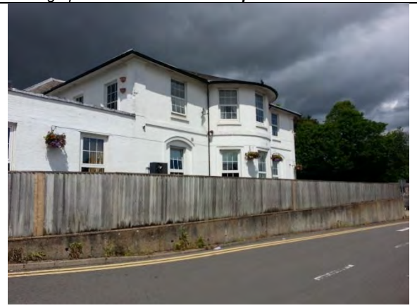
Photograph 12. TN7 – Winchester Conservative Club, south-eastern aspect.
