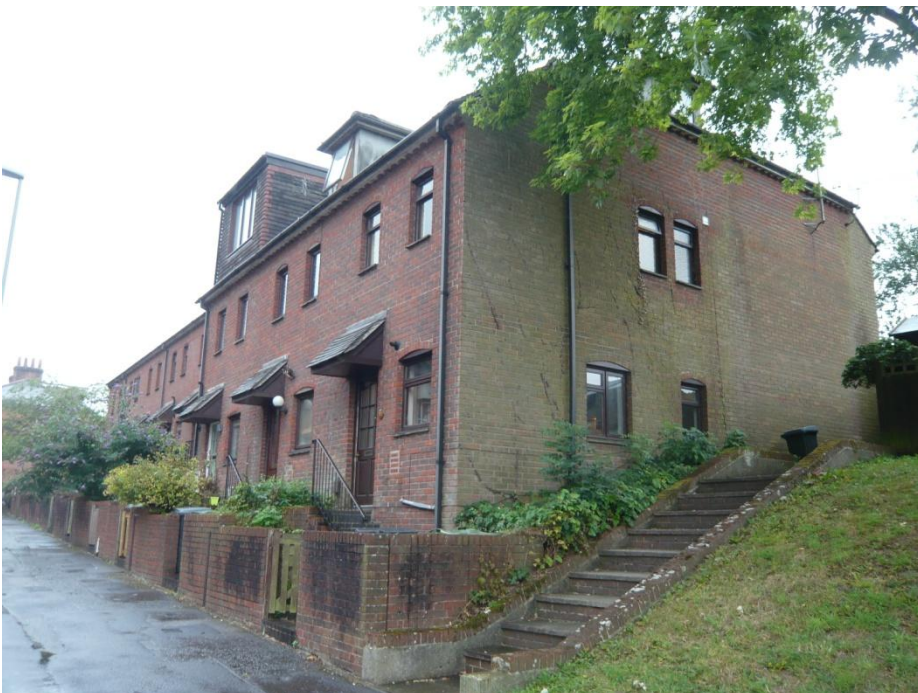
Fig.20 Terrace on the west side of Sussex Street
