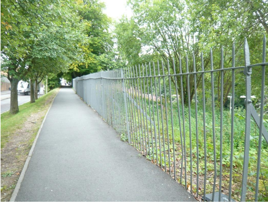
Fig.16 Wrought iron railings to the south of the station building
