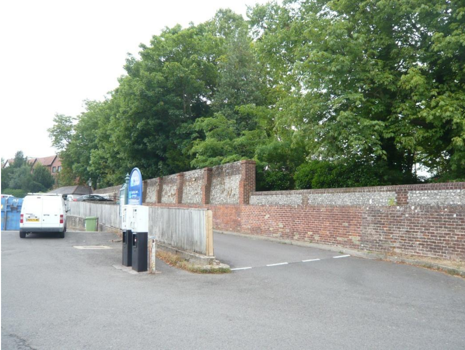
Fig.34 Brick and flint boundary walls on the south side of the Worthy Lane site
