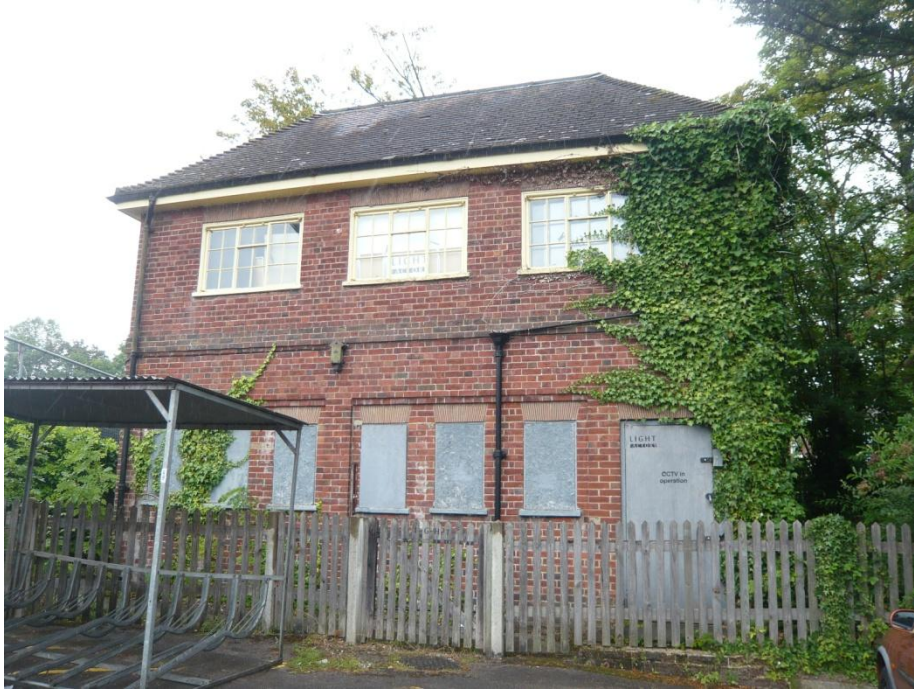
Fig.31 Former public convenience block on the Cattle Market site
