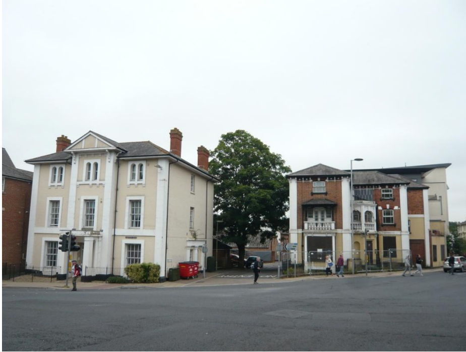
Fig.27 Former Eagle Hotel (left) and building opposite at the junction of Swan Lane
