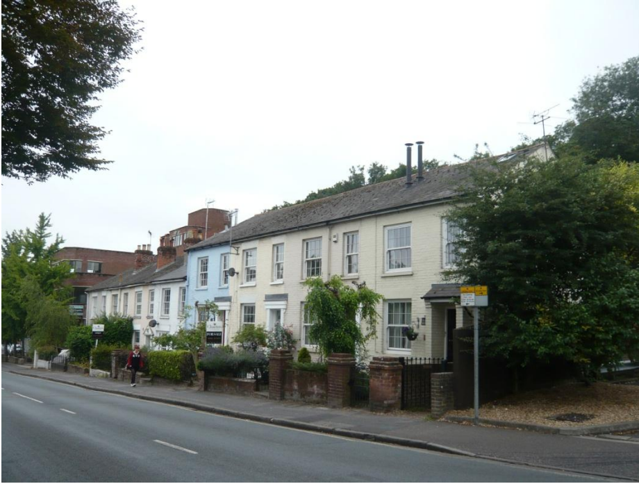
Fig.28 Victorian terrace on the west side of Andover Road Site C
