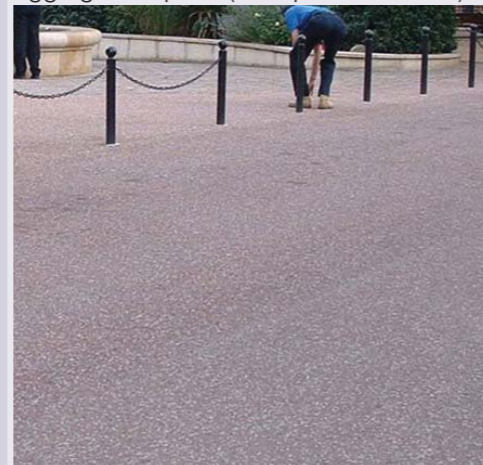
Bituminous decorative exposed aggregate asphalt (Dexapave or similar)
