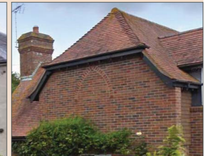
Half-Hipped roof in Cheriton
