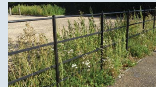
Plant Farm area - Simple iron fencing to public frontages of properties
