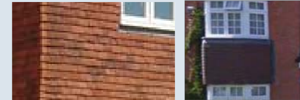
Tile hanging: High quality hanging tiles used to highlight features such as bays and dormers
