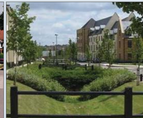
Sustainable urban drainage system, Upton
