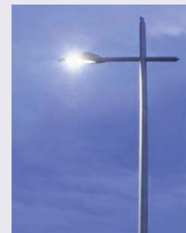
Street lighting - columns
