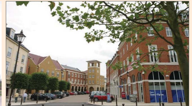
ILLUSTRATION OF USE AND ACTIVITY: Dickens Heath, Solihull. Ground floor retail/ commercial with residential above. Natural surveillance provided of public space.
