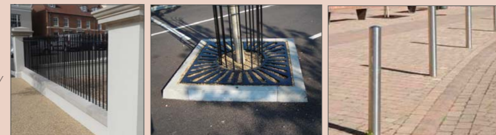
Metal street furniture, including railings to key frontages, tree grilles within courtyards and stainless steel bollards
