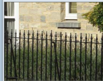
Metal railings to front property boundaries
