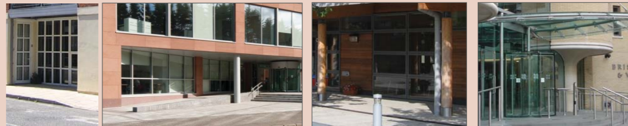
Doors should use high quality materials, often recessed or under porch feature
