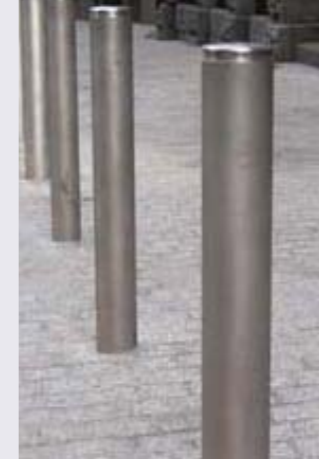
Bollards - stainless steel (Commercial Streets)
