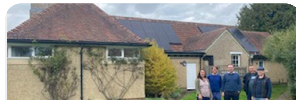
Solar panelling for Victoria Hall Sutton Scotney
