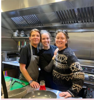
Energy efficient ventilation for South Downs Social
