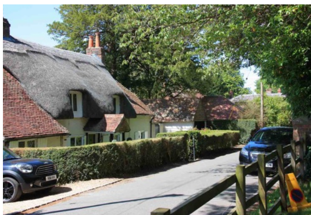
Photo 24. Little Croft on Church Street showing a variety of traditional building materials including thatch, clay plain roof and wall tiles. painted brick, and timber boarding.
