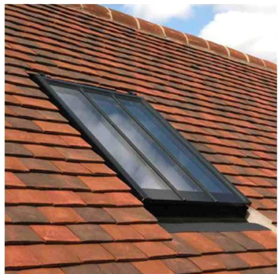
Photo 35. Conservation type skylight flush with roof surface
