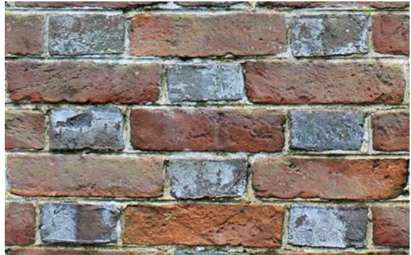
Photo 30. Brickwork in Flemish bond with red brick stretchers and grey/blue burnt headers seen on Upham Church and the Manor House and others.
