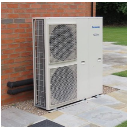
Photo 41. Air source heat pump (note the external pipework can also be visually unattractive and should be positioned carefully).
