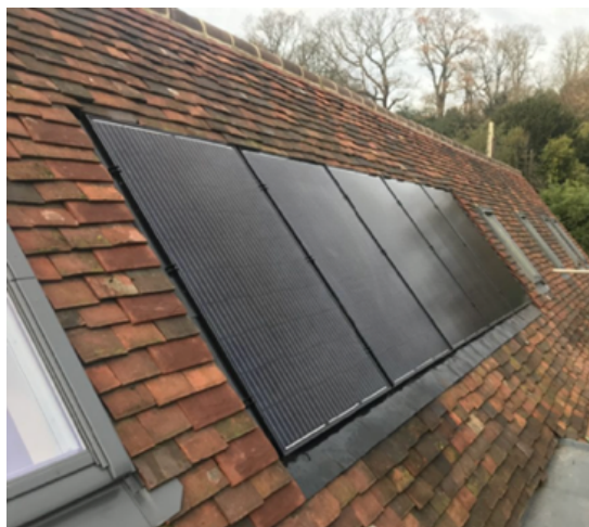
Photo 42. Solar Photovoltaic panels in a regular pattern and recessed into roof tiles.
