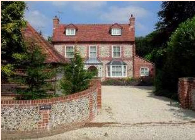
This building in Hambledon combines a neo-classical approach with Victorian style additions in the form of bay windows.
