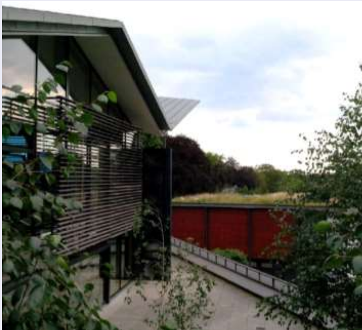
Good example of sustainable design at Winchester University, including triple glazing, louvers and a green roof.
