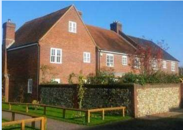
In this example in East Meon the boundary treatment has been designed in such a manner as to compliment the overall design concept for the site and the local context,
