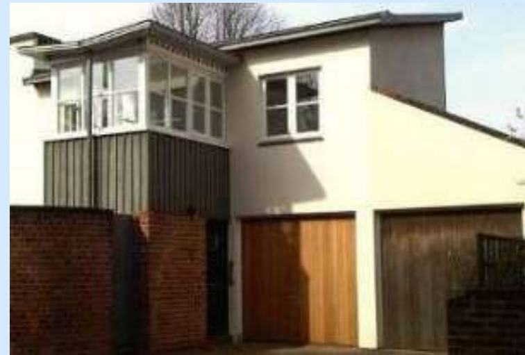
This is an example of the successful incorporation of an integral garage at this high quality development in Winchester. The garages are to the side so as to minimise the overall impact on the design of the buildings.
