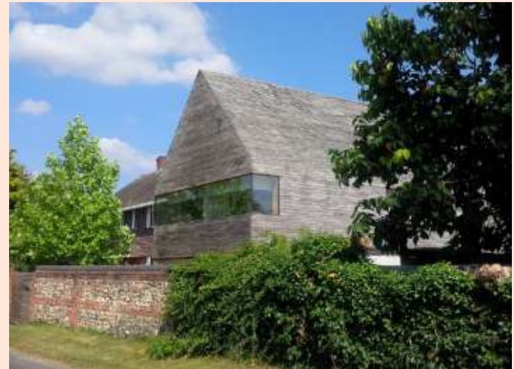
This building in Longstock in the Test Valley reinterprets the traditional rural roof form in a contemporary manner, creating a distinctive shape, reinforced by secret gutters.
