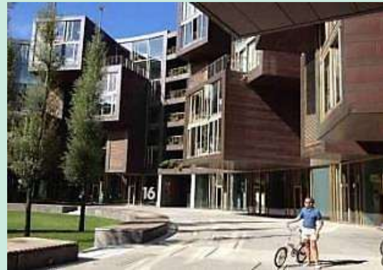
This development in Copenhagen (Tietgen Dormitories) demonstrates the significant effect of shape on the quality of spaces, creating enclosure, enriching the pedestrian experience, providing an intimate and dramatic space.
