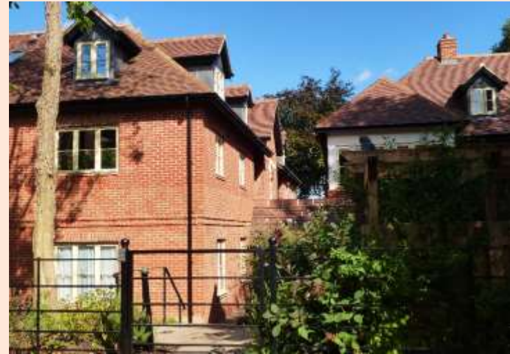
These dormers on the Milesdown development in Winchester are elegantly proportioned and well related to the rest of the fenestration. The materials and detailing are also high quality.
