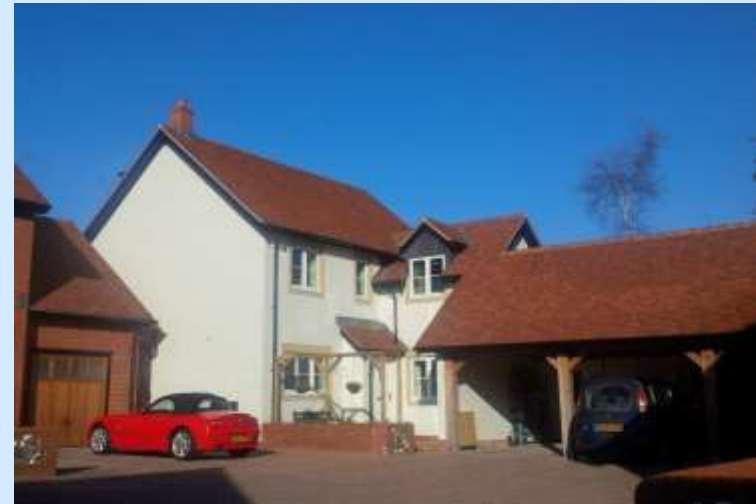
In this example from Hambledon the parking has been provided to the side of the buildings, which reduces its impact on the public realm. The car port has also been designed in a high quality traditional manner, to compliment the overall design ethos for the development.
