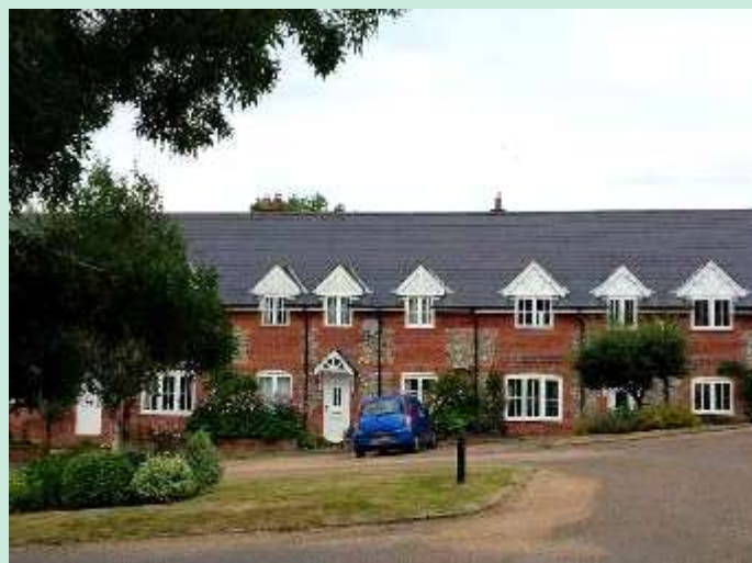
This is an example of a high quality rural development in Old Alresford, with a simple, clear layout, based on a courtyard arrangement.
