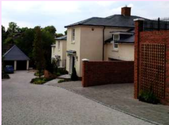
This example on Chilbolton Avenue utilises high quality paviors and subtle differences between the paving materials creating a textured finish and a successful overall composition.
