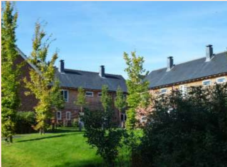
In this example in Littleton, the vertical chimney features enliven what would otherwise be a un-dynamic roofline
