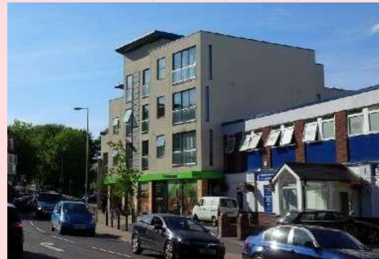
Mixed-use high density development on City Road, which utilises the highly sustainable nature of the location.
