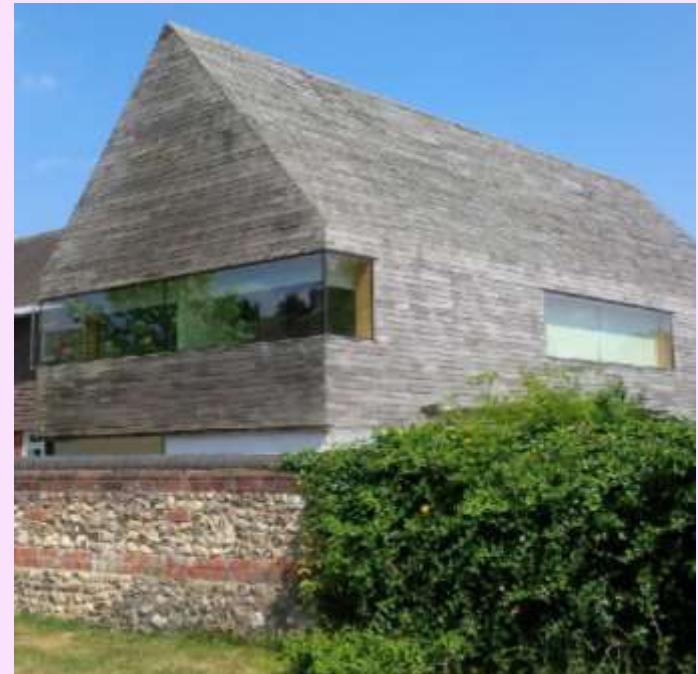
This timber cladding used on a building in Longstock in the Test Valley has weathered gracefully to silver, resulting in subtle gradations of colour.
