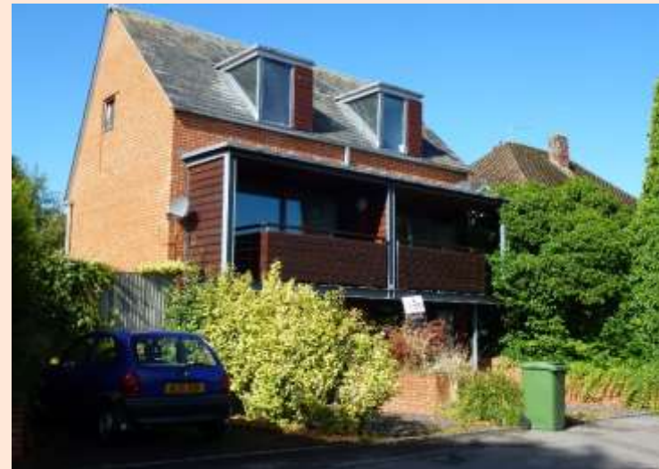
These dormers positively reinforce the overall design ethos, with their contemporary character, and crisp, high quality detailing and materials.
