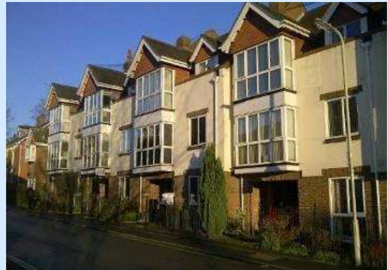
This is a good example of undercroft parking. The parking spaces have a minimal impact on the overall composition allowing for a successful relationship with the street.
