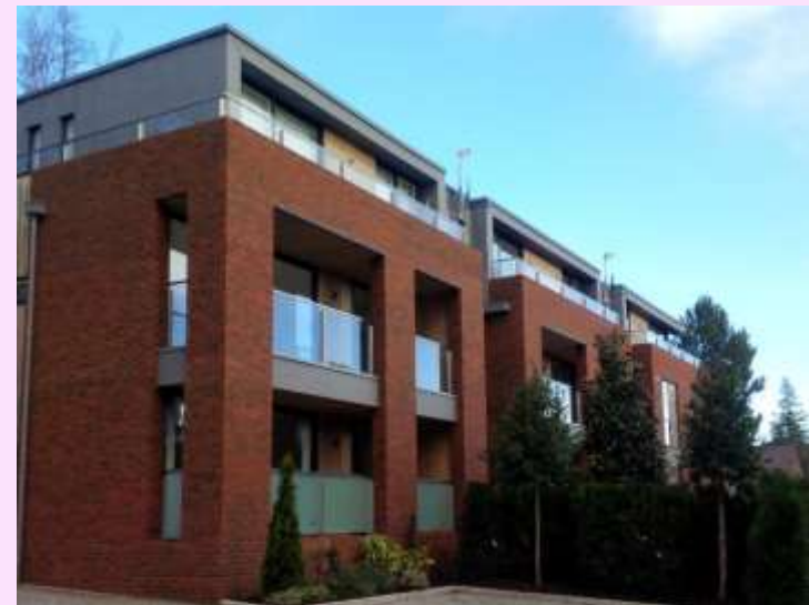
This development in Winchester utilises high quality stock bricks, well detailed balconies and a subtle blend of traditional and contemporary materials.
