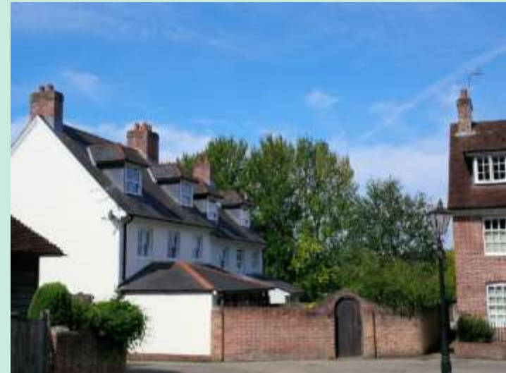
Example of a well enclosed private amenity space in a development in Twyford.
