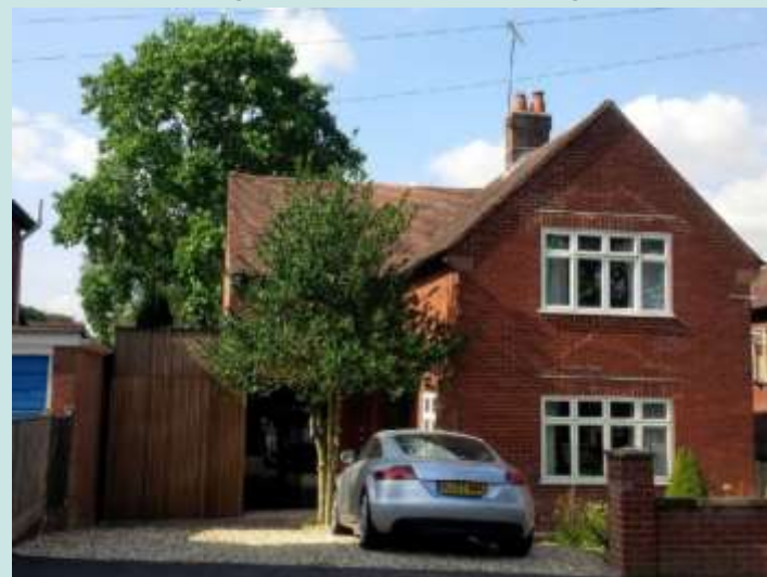
This single storey extension is sensitively related to the host dwelling, with the modest scale facilitating the subtle juxtaposition with the existing building.
