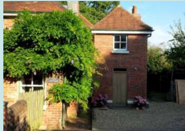
This side extension in Durley is very sensitive to the host dwelling and street scene, owing to the scale, proportions and degree of set back from the frontage.
