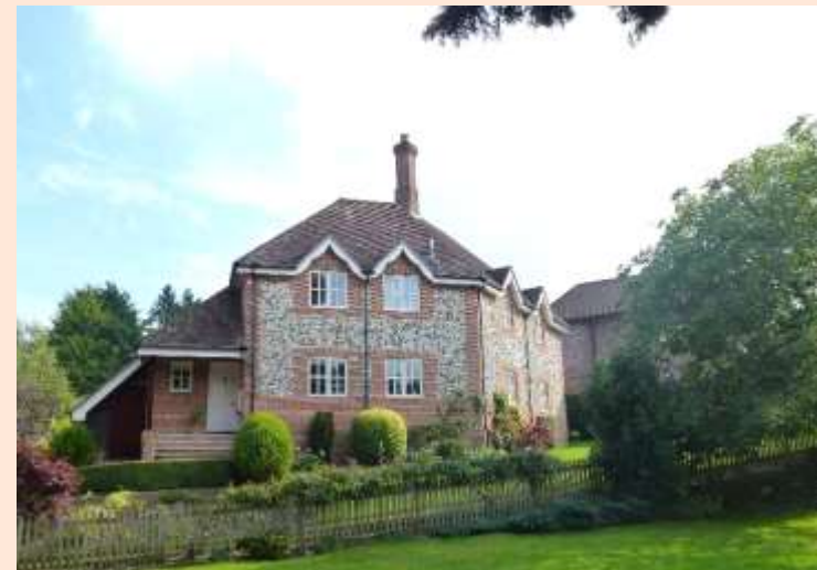
This example in Avington successfully addresses two frontages, through the form of the building and the fenestration. This has been individually designed to address the corner, as opposed to using a standard plan form.
