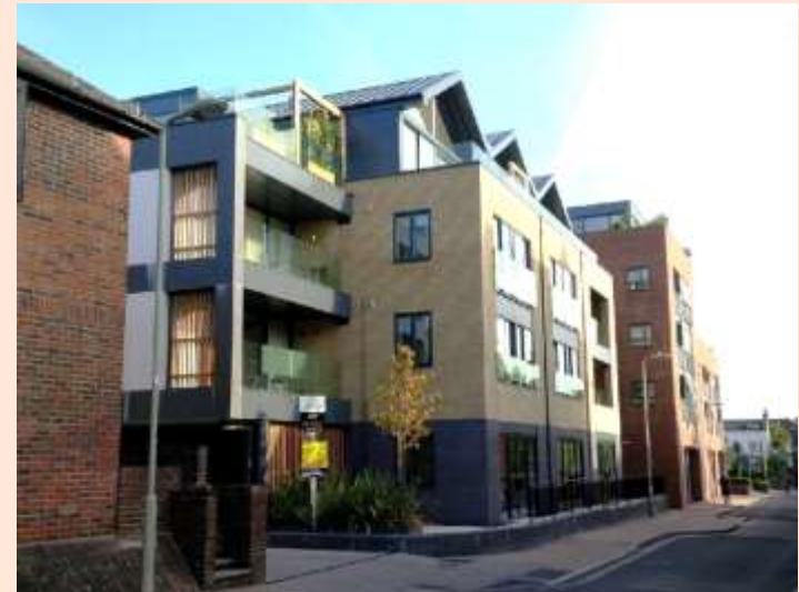
The set back top storey in this example incorporates a pitched roof form, which has been carefully designed to give the building rhythm and an elegant meeting with the sky.
