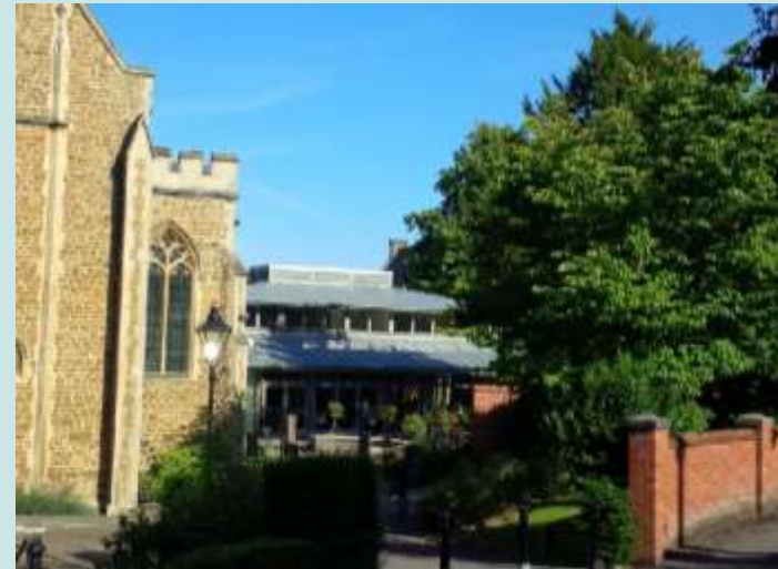
This extension to St Peters Church in Winchester utilises a high quality design, offering a subtle juxtaposition with the listed building, and enhances the character of the area.
