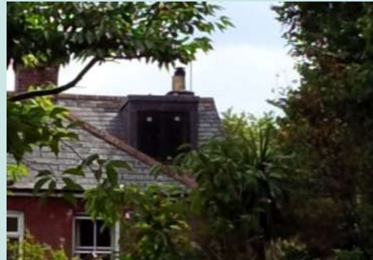
This dormer window in Hyde is well related to the existing property in terms of scale, and the use of dark grey materials allows for a successful relationship with the existing slate roof.
