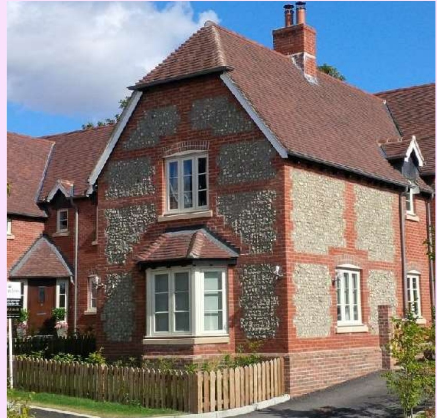
This flint walling in Cheriton is also successful, giving a textured, traditional appearance. The brick quoins also play a significant role in the success of the finish achieved.
