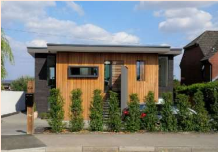
This example employs a contemporary approach to the fenestration in terms of shape, size, arrangement, materials and detailing
