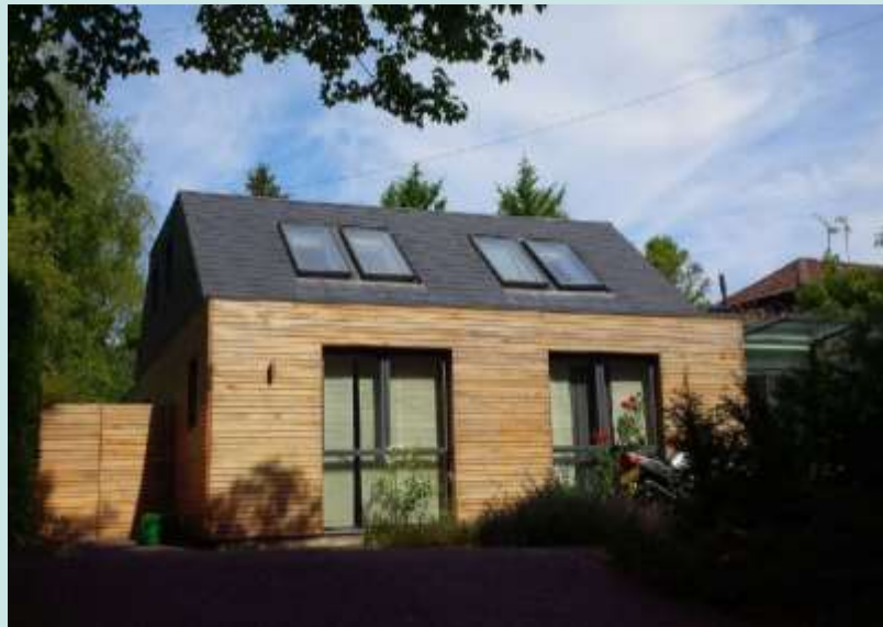
This roof extension successfully minimises the scale of the extension, whilst the rooflights are well related to the fenestration.
