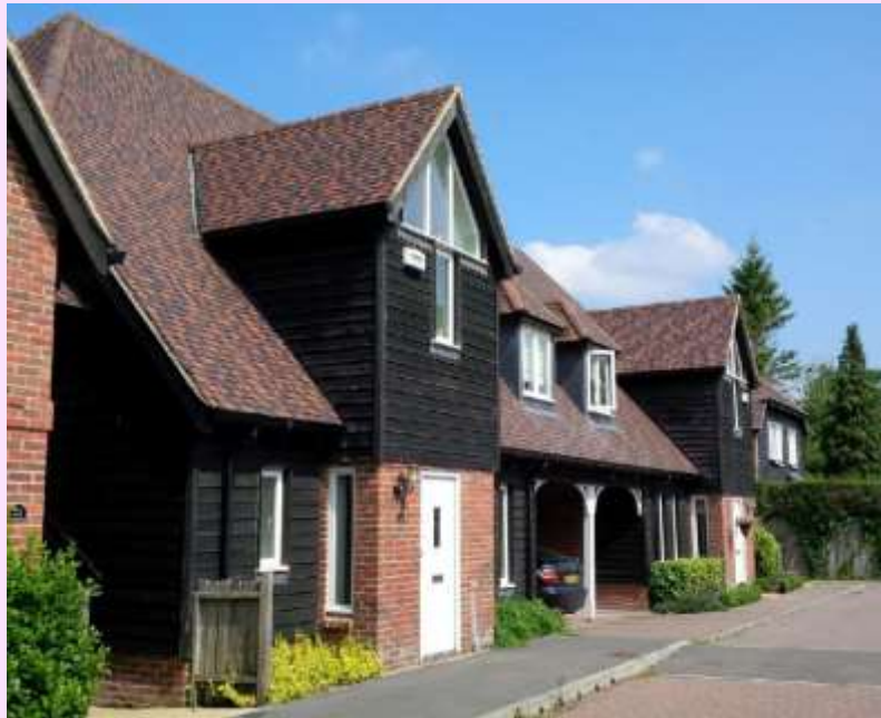
This development in Corehampton utilises stained cladding in order to reflect the local rural vernacular, reinforcing the sense of place.
