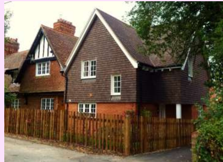
High quality traditional materials and detailing in Micheldever Station, with open eaves, recessed windows and textured clay tiles.
