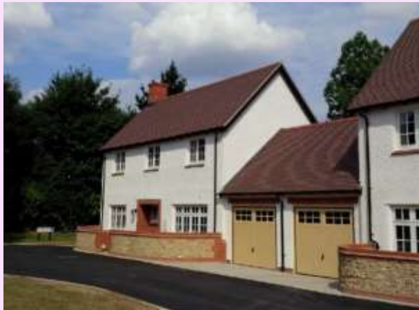
The Francis Gardens site in Winchester utilises rough render, giving an attractive traditional appearance
