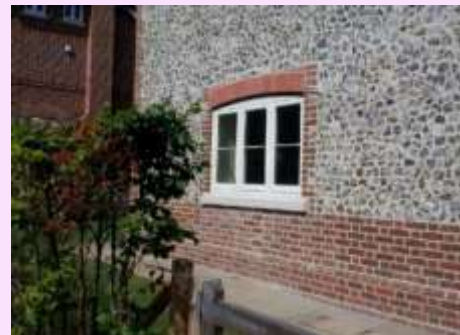
This flint walling in Cheriton is also successful, giving a textured, traditional appearance. The brick quoins also play a significant role in the success of the finish achieved.
