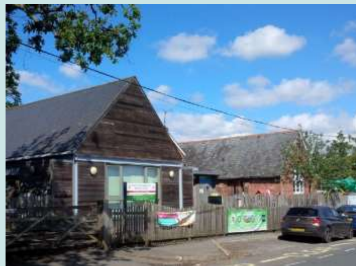
This extension near Newtown has been sensitively related to the host building in terms of form and scale, with the contrasting material reflecting the transition of the building form.
