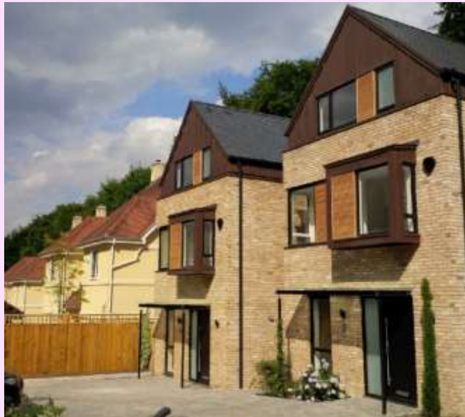
This scheme on Chilbolton Avenue utilises high quality, durable window materials and detailing by using powder coated aluminium in a colour that contrasts with the buff brick.
