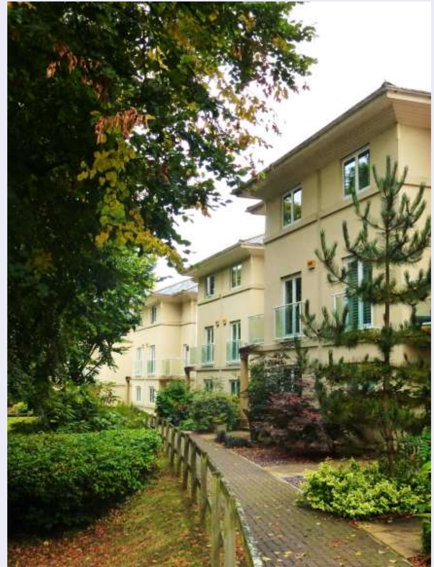
Example of a combination of key urban design principles in Winchester, with good enclosure, active frontages and a well overlooked footpath.
