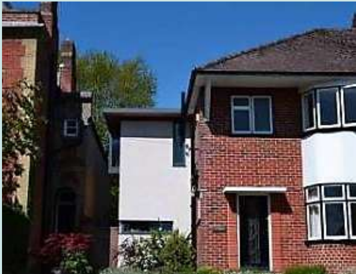
This extension in St Cross (Edgar Road) is elegantly proportioned, both in terms of the extension itself, but also in relation to the host dwelling. The extension is set back and is well related to the host dwelling in terms of eaves line.
