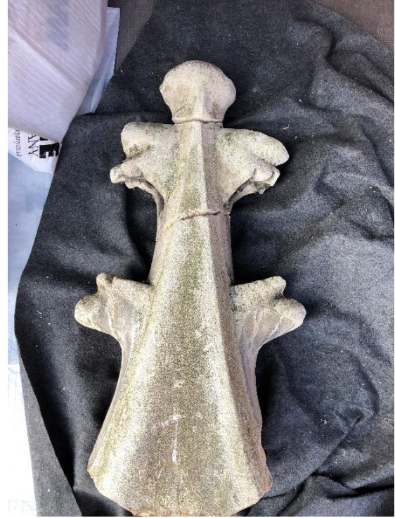
Fig 17 – Rear of assembled finial
