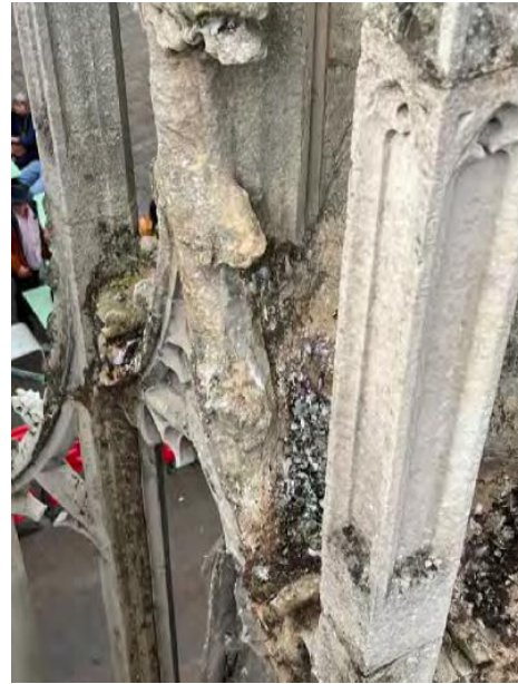
Fig 26 – Waterways between stage 3 and 4 statues.
