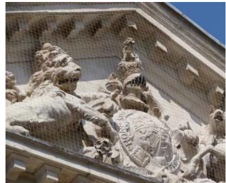
Fig 28 – netting on a historic building
