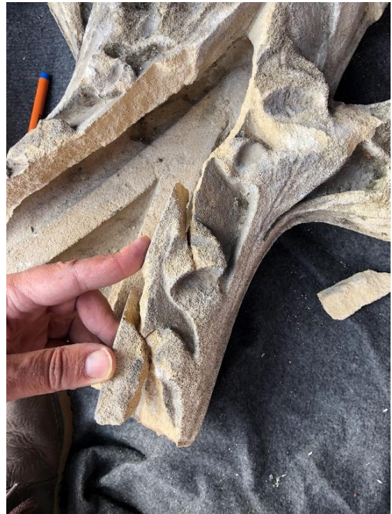
Fig 18 & 19 – reassembled fragments from the base of the finial.
