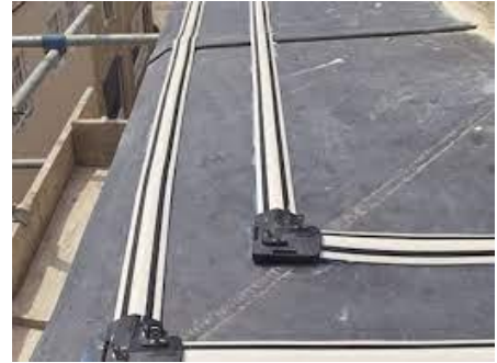
Fig 30 – bird shock tracks.
