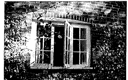
Timber casement with mullions
