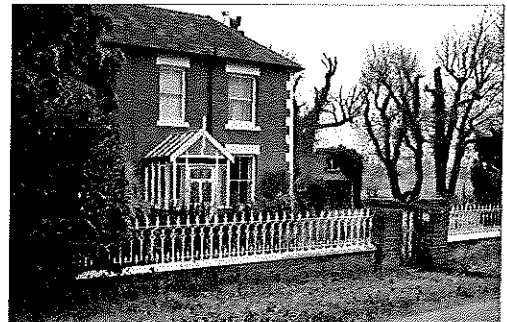
House in Ingoldfield Lane
