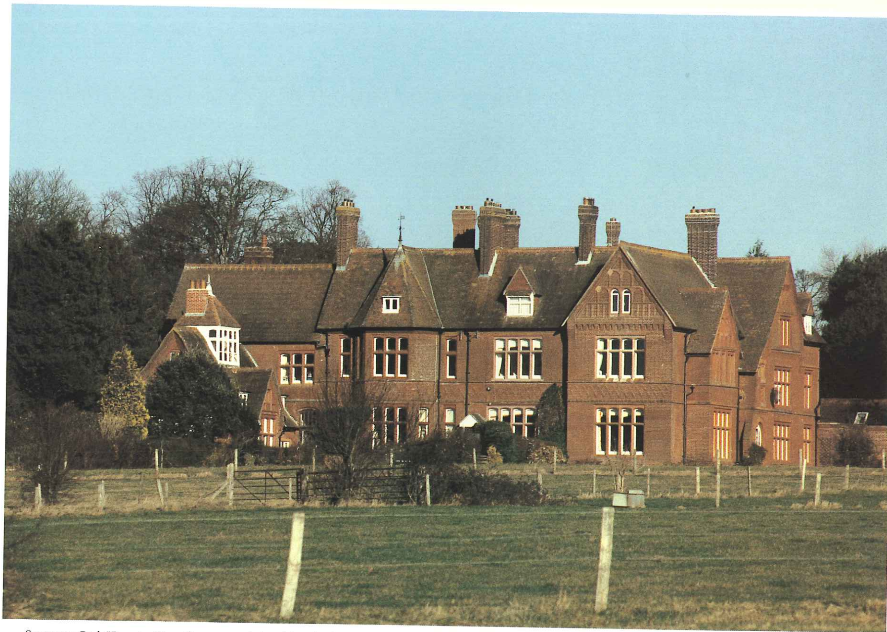
Swanmore Park House in Upper Swanmore: designed for Charles Myers by Alfred Waterhouse RA (architect of London's Natural History Museum) it was completed in 1880.
