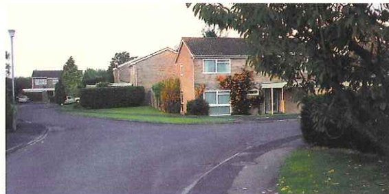
Detached 1970s houses in Crofton Way.
