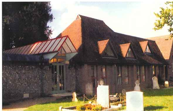
The Paterson Centre, in Church Road.
