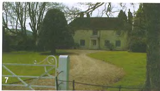
7. Borough Farm House, Sloe Lane, 18th century
