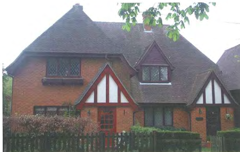
Photographs of new housing at New Road, Brunel Close and Andover Road Micheldever Station
