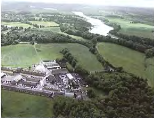
Bury Farm Industrial Estate with the River Hamble in the background
