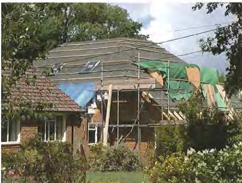
Building work in progress at Curdridge Lane
