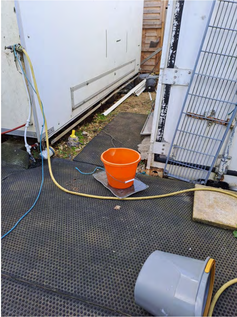
Rear of butcher's shop to left, walk-in butcher's freezer to right
