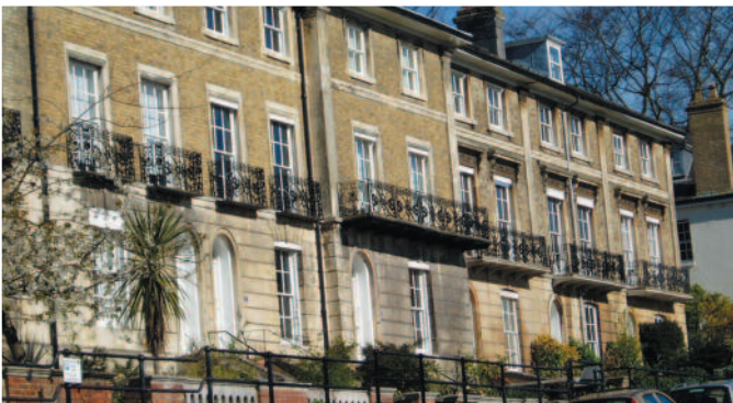
Clifton Terrace - the first development
