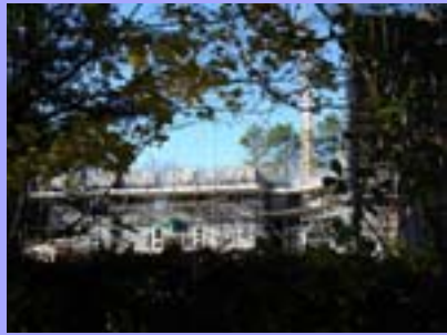
Demolition and redevelopment - King's Crescent
