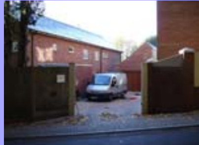
Redevelopment at Dawnhill 2
