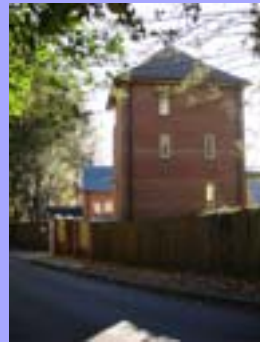
Redevelopment at Dawnhill 1
