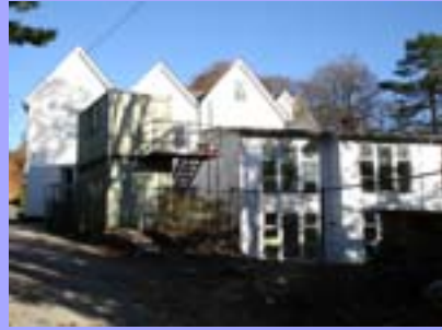
Extension of existing building - Westacre Nursing Home
