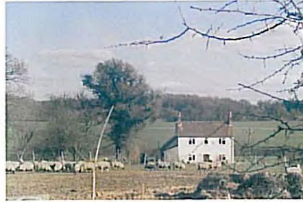
Pounds Farmhouse, Trampers Lane
