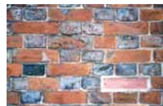
Wrong Mortar used in repair
