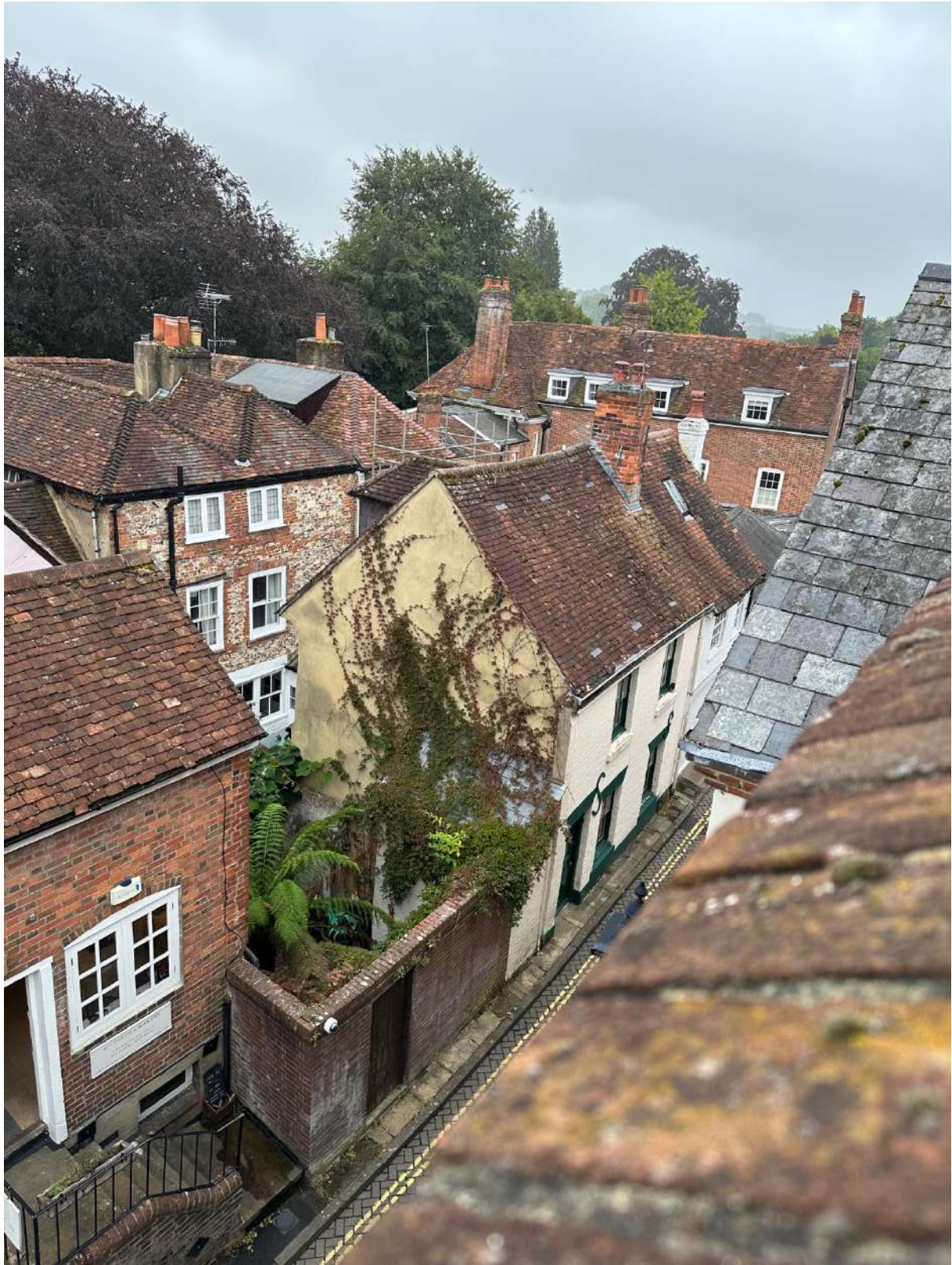
Fig D14: View from 2 Calpe Yard Terrace, north east
