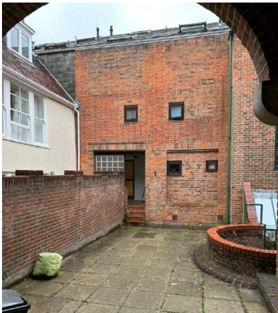
Fig D2: 2 Calpe Yard, Western showing ground floor garaging
