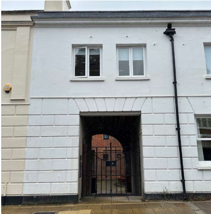
Fig D1: Entrance to Calpe Yard from St Thomas St
