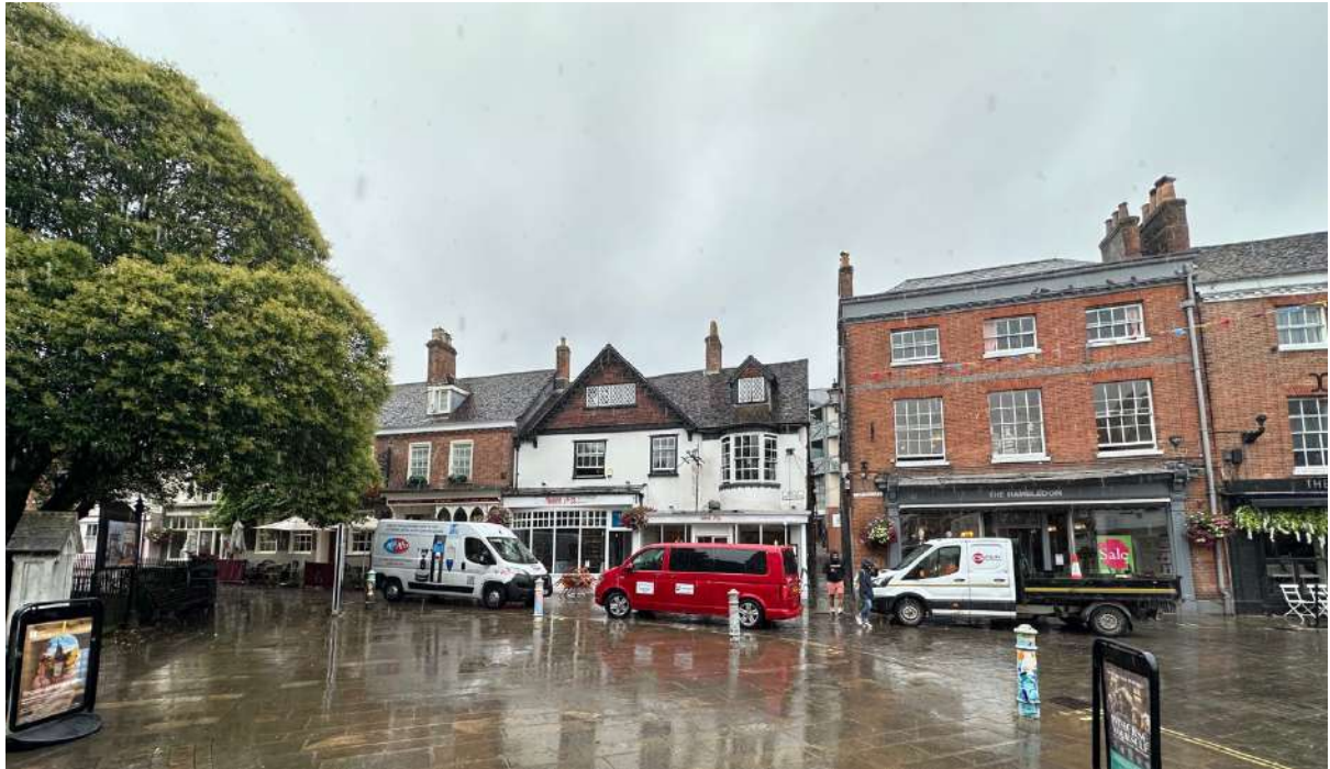
Fig D7: View towards Calpe Yard (behind white rendered building) from The Square / Great Minster Street
