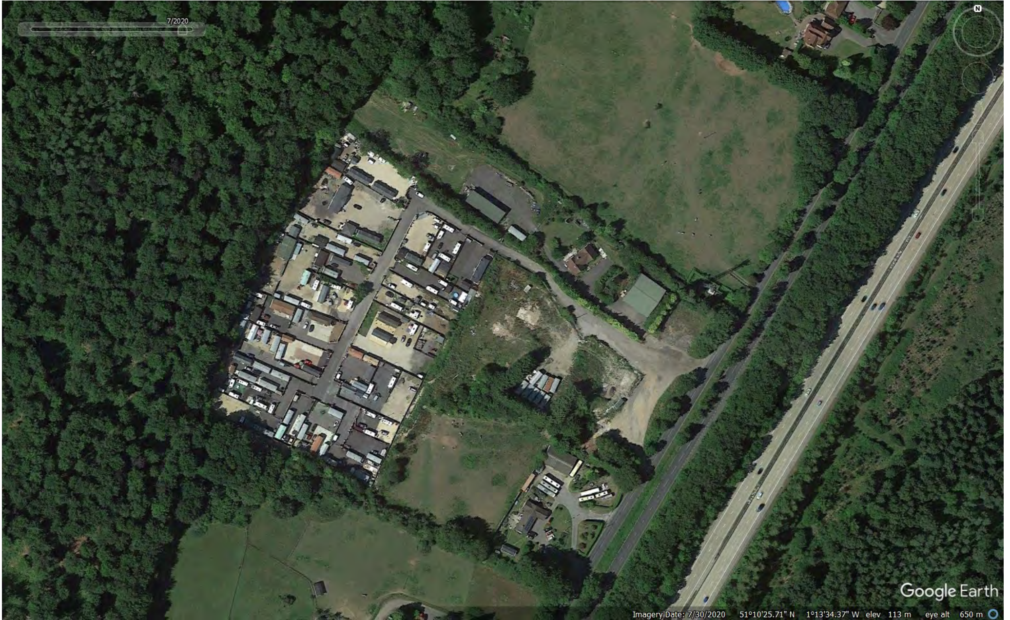
Aerial Image Dated 30/07/2020
