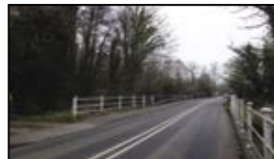
B3335 Highbridge Rd River Bridge
