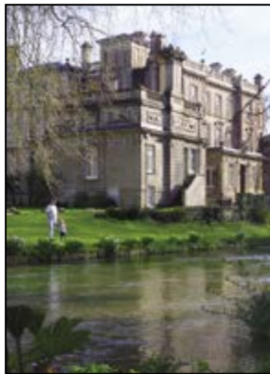
Brambridge House, Kiln Lane
