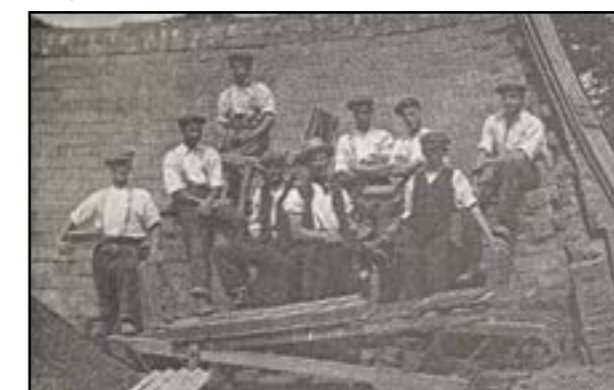
Phillips Brick Works c.1840s
