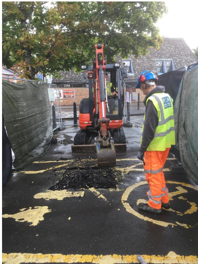
Excavating a test pit for BH01 (PCA)
