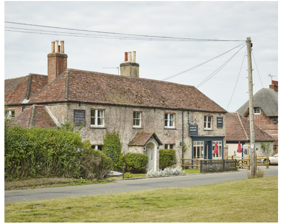
Northbrook Arms, East Stratton
