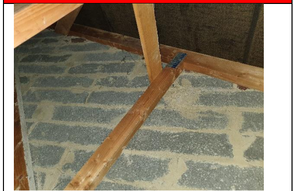
6. View into roof void
