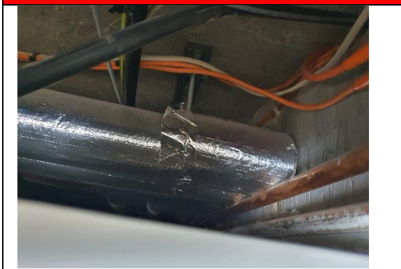
5. View above g/f ceiling
