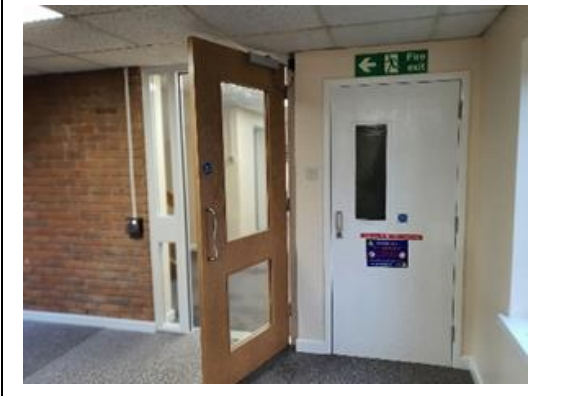
7. Main door between wings dragging on carpet
