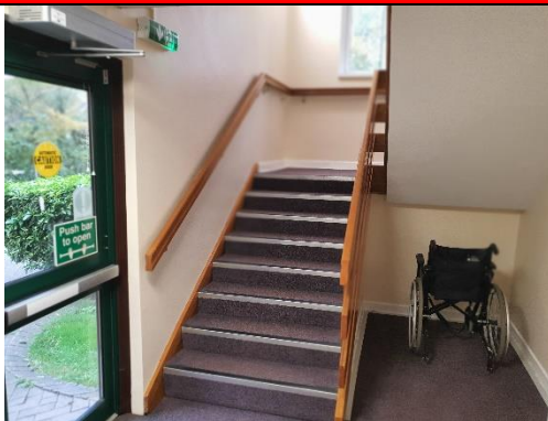
3. Wheelchair at base of stair in zone 3
