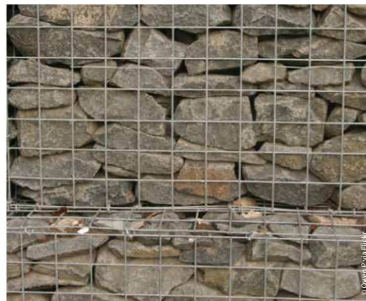
GABION BASKETS HOLDING SITE-WON MATERIAL
