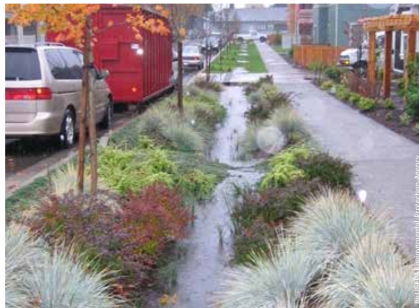
PLANTED SWALE FILTERING & ATTENUATING WATER
