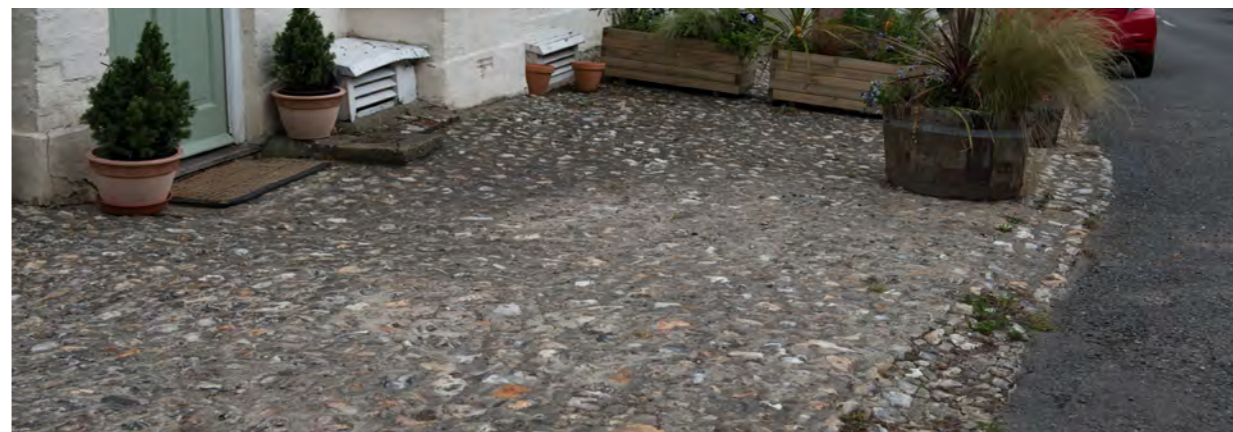
Top: flint cobbled road margin, High Street
