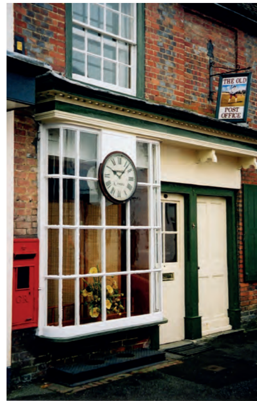
Top: The Old Post Office, West Street
