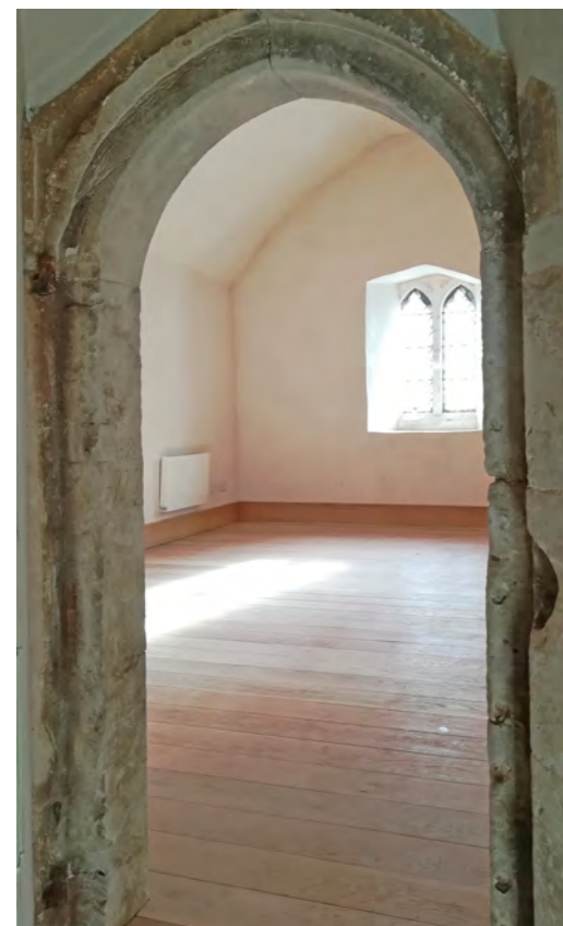
Left: the newly-created room above the south porch of the church.
