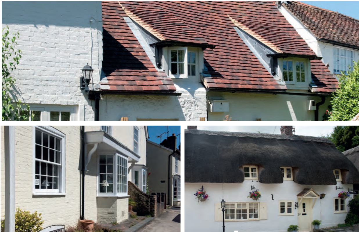
Top: Dormer windows on Green Lane Top and above left: Approved slimline double glazing in listed buildings. Above left: Sliding sash and bay windows on East Street Above right: Thatched cottage, Rosemead
