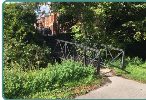
Existing bridge with stepped access to Monks Road
