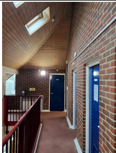
11. 1 st floor SD/rooflights and store door
