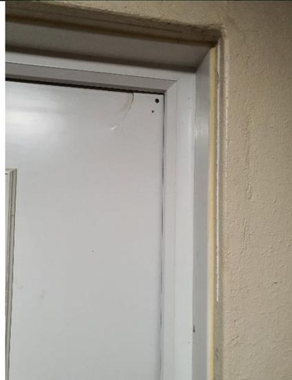
17. 1<sup>st</sup> floor stair door, 10mm gaps, 12mm overhang
