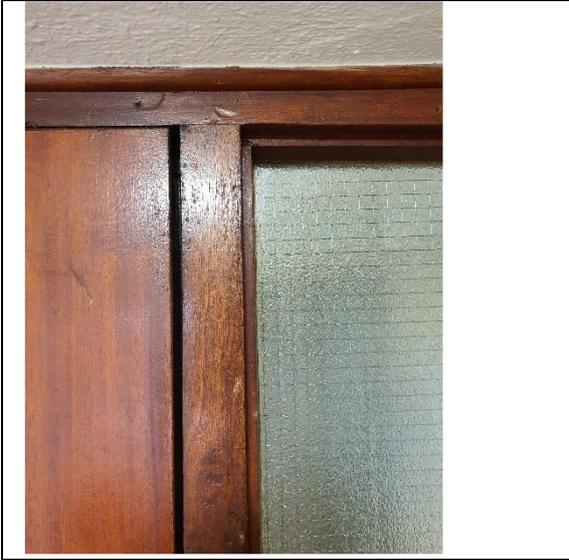
10. 3<sup>rd</sup> floor corridor door – 10mm overhang and 10mm gaps
