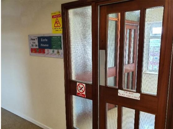
6. 6<sup>th</sup> floor stair door warped (15mm)
