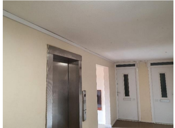
2. Example of cables in plastic trunking
