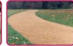
Perimeter track of self-binding gravel for a natural appearance
