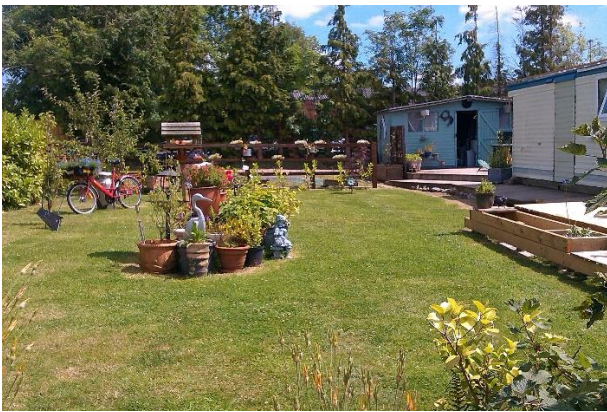
Photo 21 taken 15.07.2014 showing garden and new decking under construction
