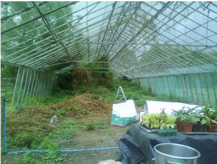
Photo 17 taken 19.07.2011 showing additional clearance works in glasshouse (105)
