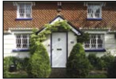
Keepers Cottage, Church Lane
