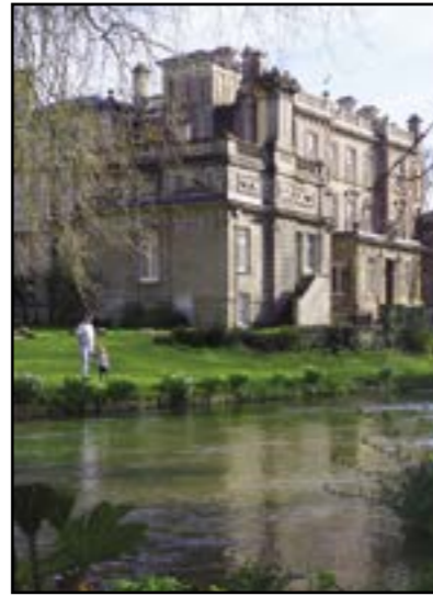
Brambridge House, Kiln Lane
