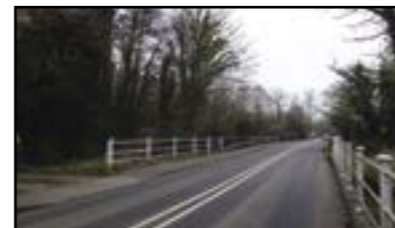
B3335 Highbridge Rd River Bridge
