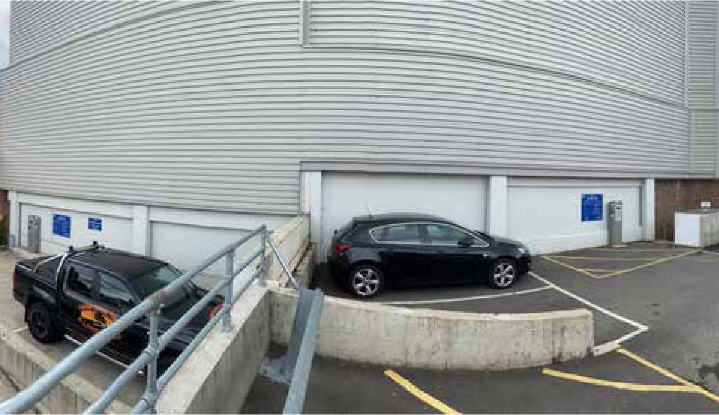
Exterior of the end of the car park – this is the ‘new’ metal end wall where they cut the old car park in half – as you can see, no entrance / exit.
