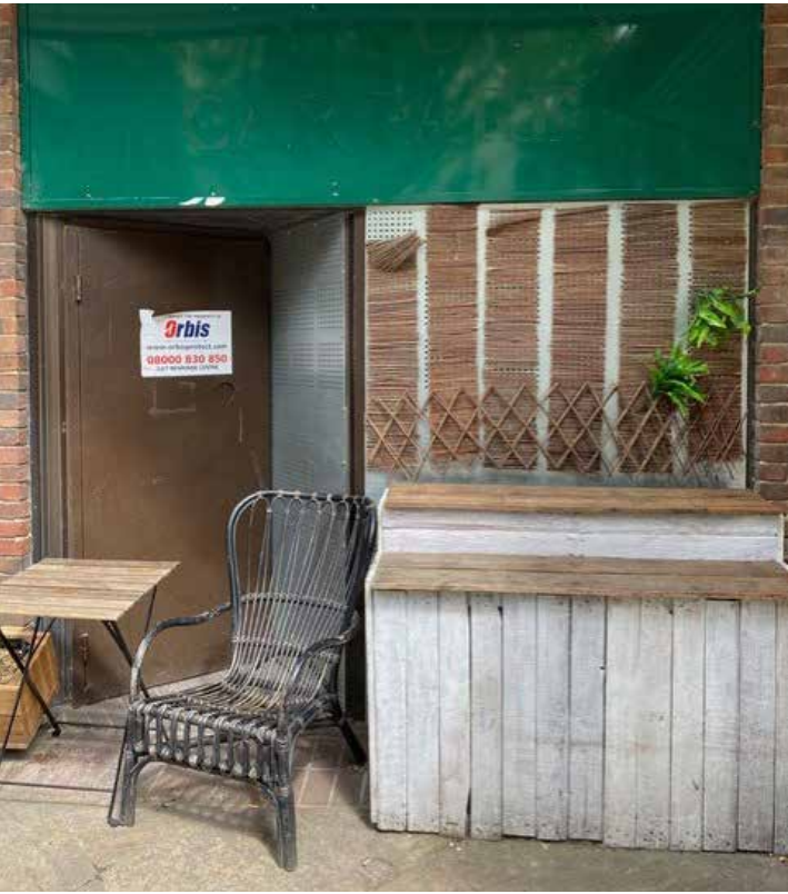
Current (and only) access via single door at ground level – possible to widen slightly, but the stairs upwards would prevent a full double door width.
