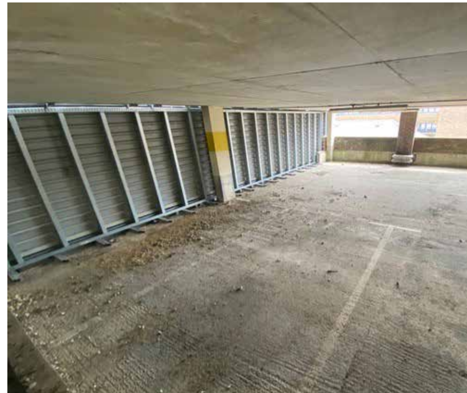
The building has been effectively sliced in two and capped with a metal wall.
