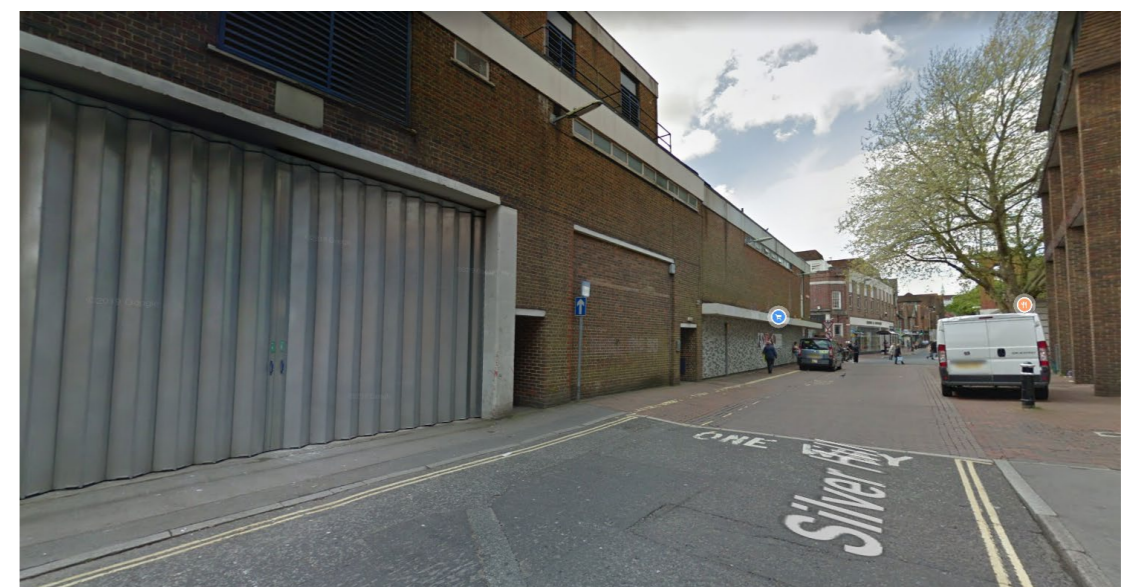
Figure 32 - Potential location for bus stops to replace taxi rank on Silver Hill (east), showing Sainsburys service yard in foreground (image from Google Streetview)
