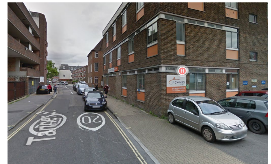
Figure 29 - Narrow footway on Tanner Street adjacent to GP Surgery (image from Google Streetview)
