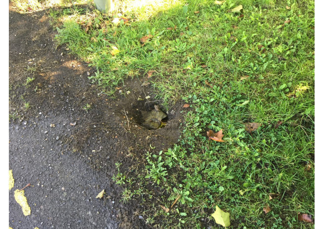
Wooden posts have rotten leaving hazardous holes in the ground
