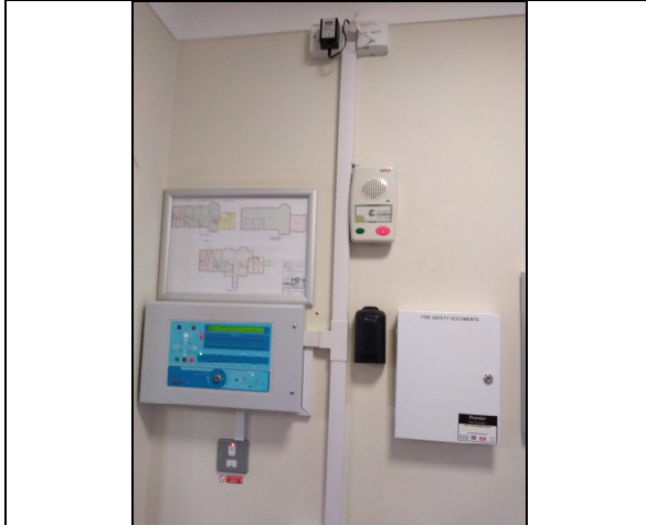
1. Fire alarm panel & Tunstall unit.
