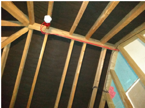
7. Smoke detector in loft void.
