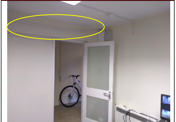
6. Loose conduit to office.
