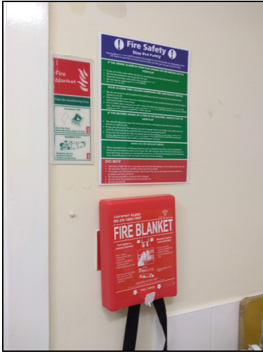
1. Fire safety signage in kitchen.
