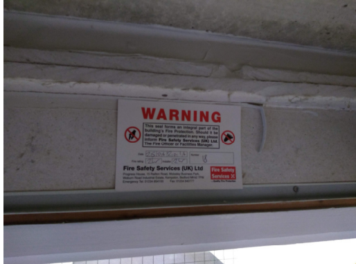
3. Fire stopping label above fire-doors.
