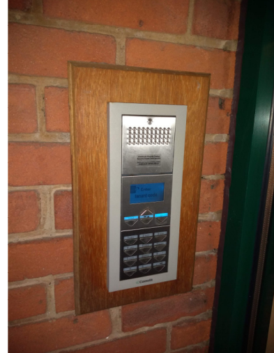
2. Front door intercom.
