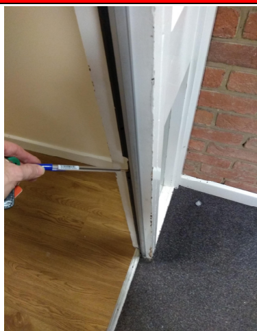
11. Damaged perimeter smoke seal.
