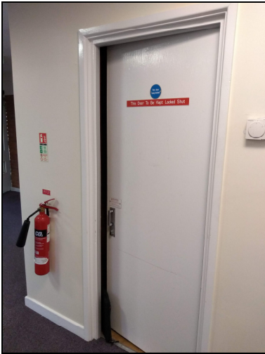
9. Boiler cupboard to reception area.
