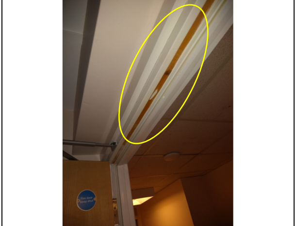
4. Missing intumescent strip: guestroom.
