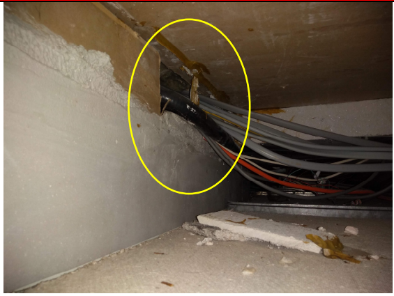
5. Break in compartment above fire doors.
