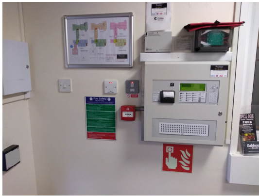
1. Fire alarm panel & zonal chart.
