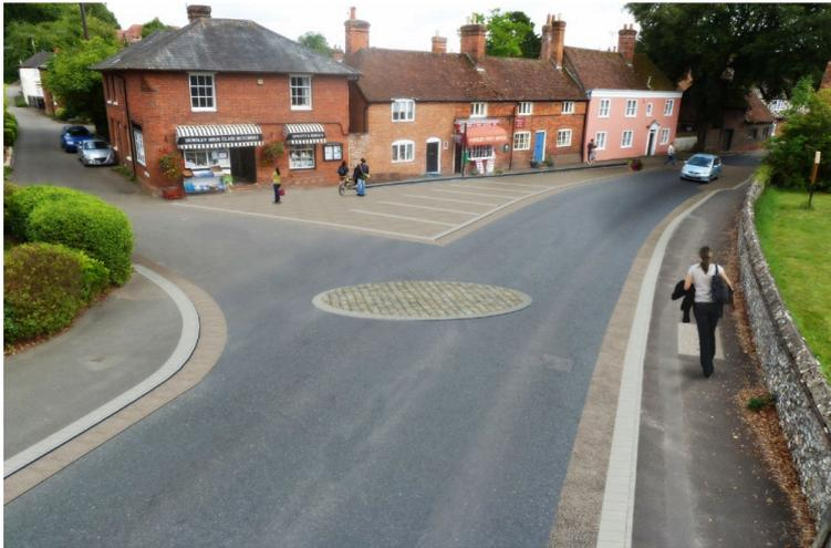
The illustration shows a drive-over roundabout and a treatment of the surface of the carriageway which is both visually interesting and attractive, as well as giving the impression that the road is narrower than it is.
