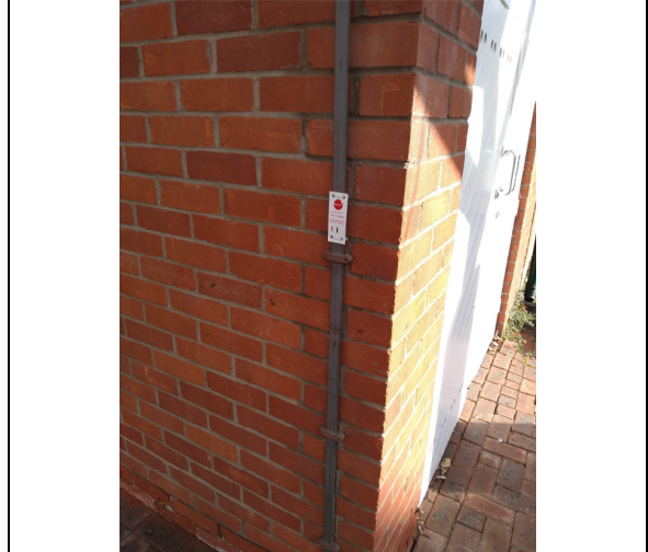
10. Lightning protection strap.
