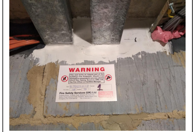
2. Fire stopping in ceiling void.
