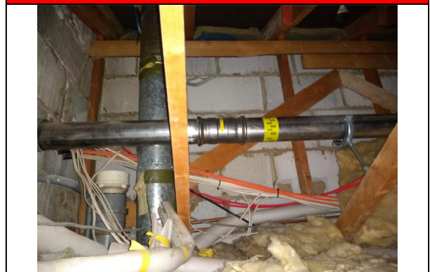
6. Gas pipe in ceiling void.
