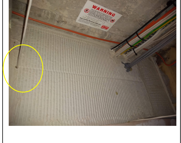
4. New cable in ceiling void.
