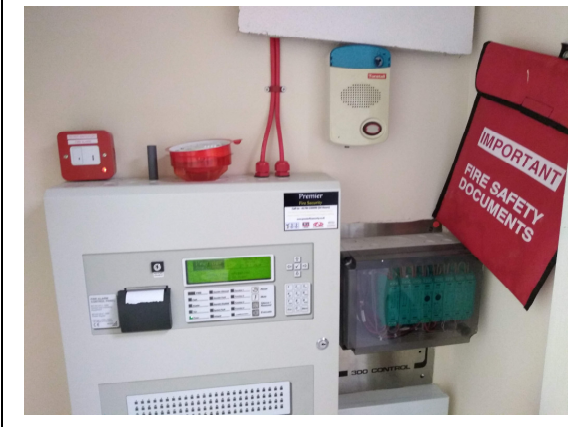
1. Fire Alarm Panel.
