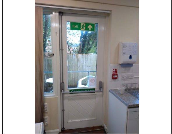
8. Main kitchen escape door.
