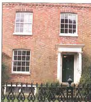
Windows should generally be small paned with both the overall window and individual panes taller than they are wide
