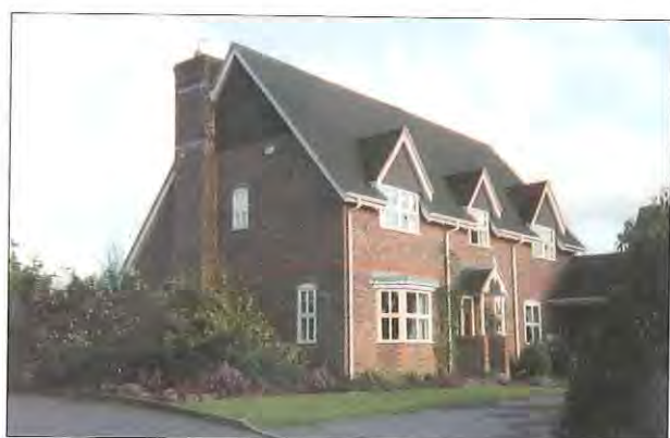
New building with small open porch and dormers
