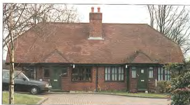
New building with half-hipped roof
