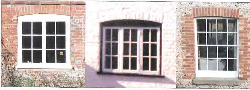
An important detail is the arched brick window head
