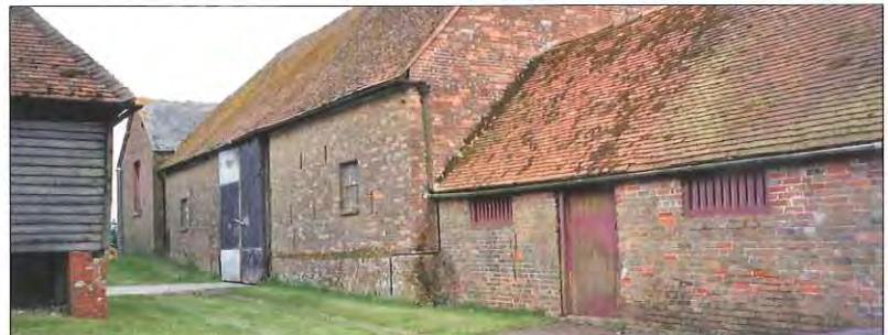
Farm buildings at Corhampton Lane Farm
