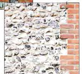
Flint and brick wall
