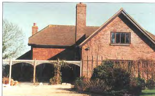
New building appears modest in scale when viewed from the road
