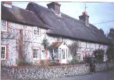
Flints are often used in houses and are common in boundary walls
