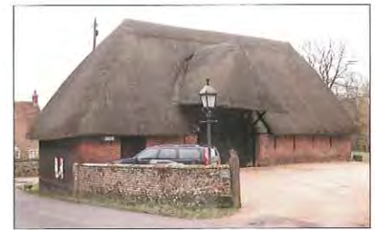
The barn in Meonstoke High Street
