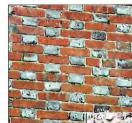
Red brick is the predominant building material, often laid in Flemish bond with burnt headers
