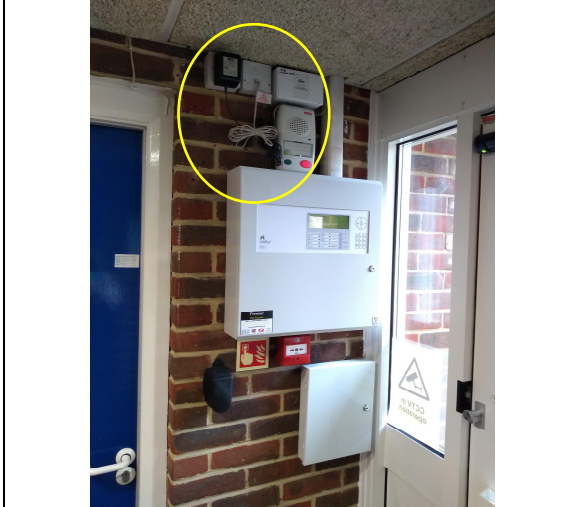
1. Fire Alarm Panel & Tunstall unit.
