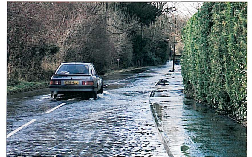
Flooding at East End, January 2001
