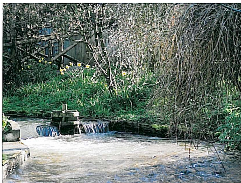
Weir at Mill House
