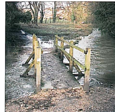
'Pooh Bridge', November 2000
