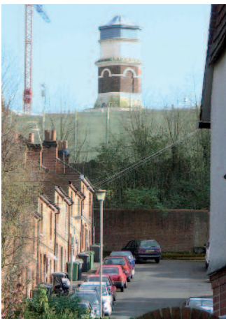
View to Greenhill Avenue and the prison
