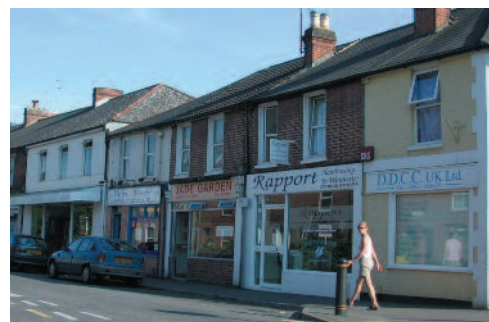
Stockbridge Road shops
