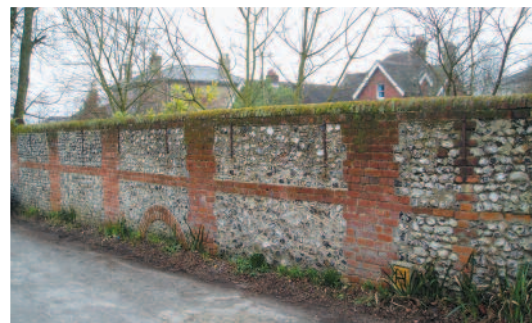
An original wall
