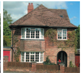
A typical facade
