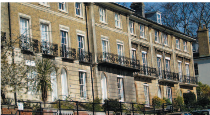
Clifton Terrace - the first development
