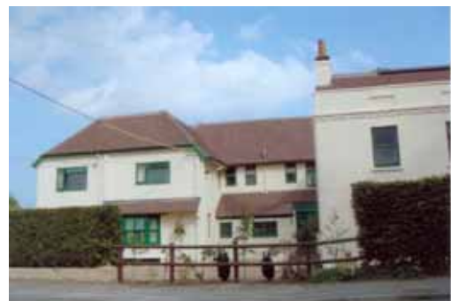
Elderfield after renovation
