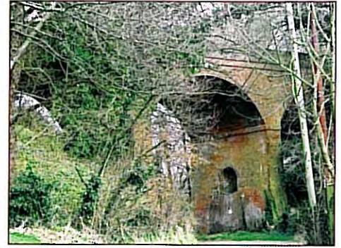
The old railway bridge over Northington Road
