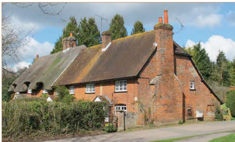
Thyme Cottage, Compton Street in foreground rear from left: Linden Cottage and Century Cottage
