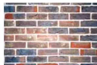
Lime Mortar Repointing
